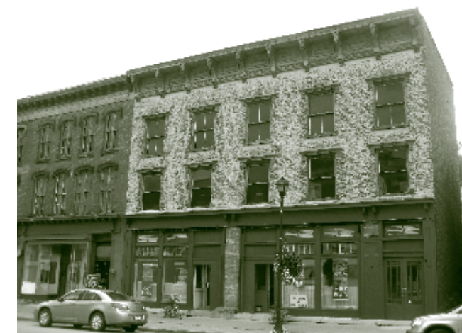
First known as Diefendorf Hall, the building at 47 Main Street was a theater in the late 19th and early 20th centuries. Later, housing the American Legion, it served as a venue for community events such as dance recitals, high school proms, public card parties, church bazaars, and fashion shows.
