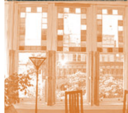
Historic wood windows were repaired and retained in the Connor's Apartments in Corning.
